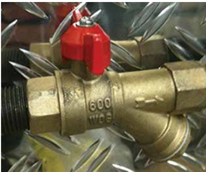
FIGURE 7-1: (STEP 1) SHUTOFF VALVE WITH STRAINER SHOWN IN THE OFF POSITION
