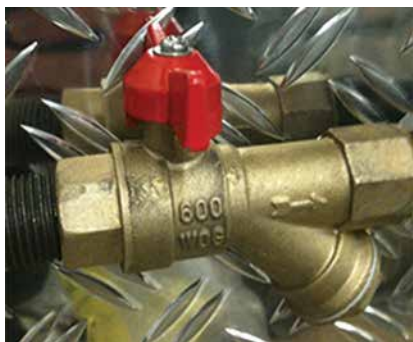
FIGURE 6-8: (STEP 9) SHUTOFF VALVE WITH STRAINER SHOWN IN THE OFF POSITION
